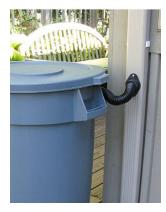
Also available are "automatic" diverters like the one I use, the "Earth Minded" kit, widely available online and at local places like Lowe's and Home Depot. This one is harder to install, although the kit is quite complete, including hole-saw bits and all the needed fittings and hoses. It probably does not capture all of the rain in the downspout.
