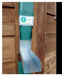
The "Save the Rain" diverter offered through Great American Rain Barrel is very easy to install and captures all the water. You just cut off the downspout, insert this square diverter to guide the water into the barrel, and reconnect the bottom of the downspout to the bottom of the diverter.
