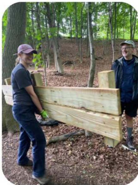
In June, volunteers helped to install a new boardwalk at Flint's pond
